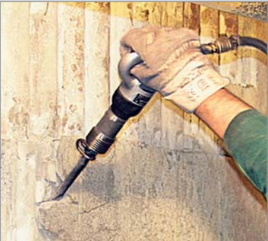
Effortless removal of plaster and tiles
